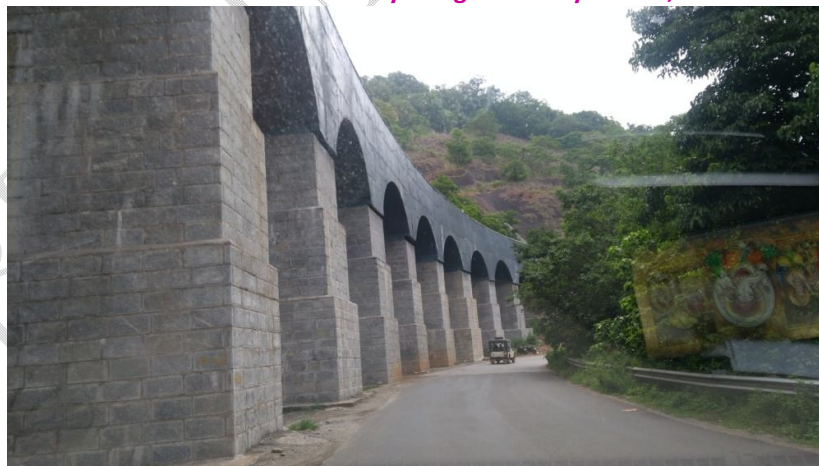
Kollam-Schenkottah Railway Bridge near Aryankavu, Kerala.
