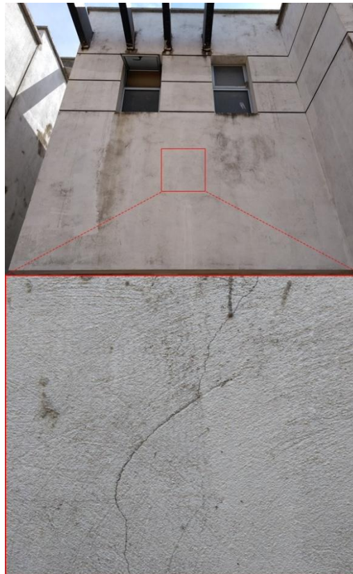
Figure 3 – Upper facade after 30 days, at the beggining of the appearance of the cracks, right side
