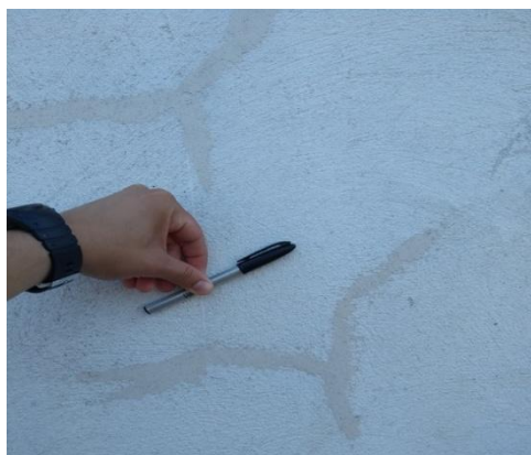
Figure 12 - Sample of cracks treated after 48 hours
