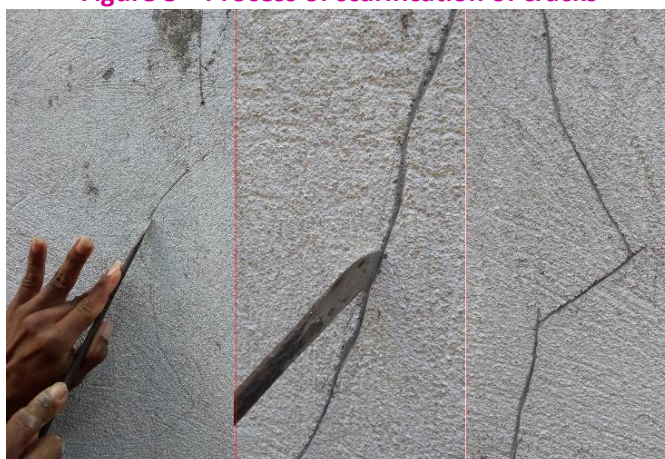
Figure 8 – Process of scarification of cracks
