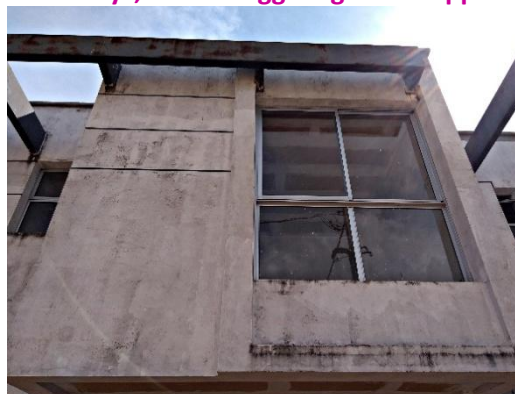
Figure 4 – Upper facade after 30 days, at the beggining of the appearance of the cracks, left side
