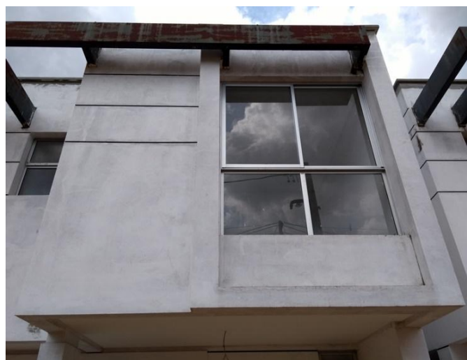
Figure 14 – View of the upper facade 48 hours after the product applied, left side
