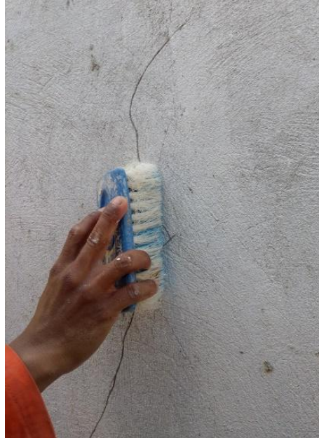
Figure 9 – Cleaning the scarification with a brush
