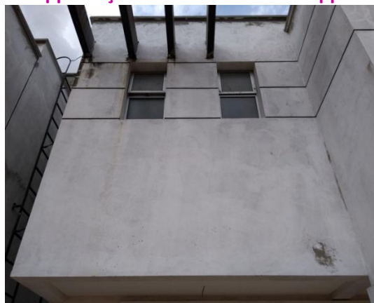
Figure 13 - View of the upper façade 48 hours after the applied product, direct side
