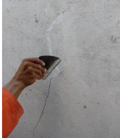
Figure 11 – Application of the product with the aid of the spatula
