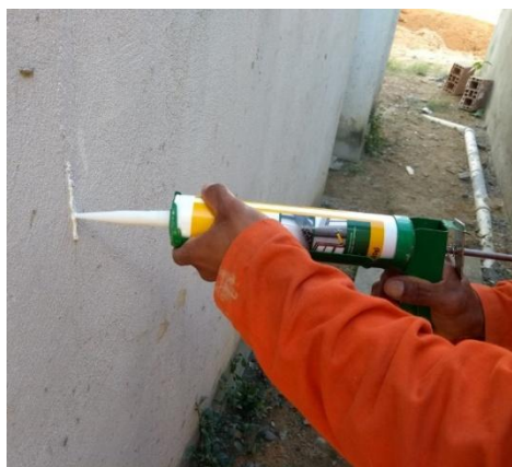
Figure 10 – Application of the product with the aid of a hand gun.
