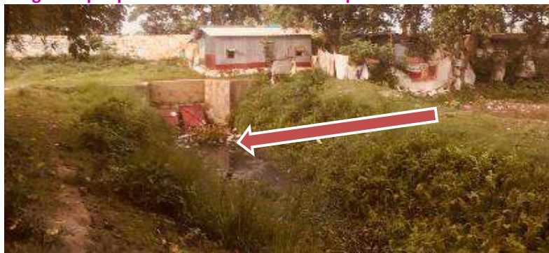
Plate 11: The gate through which urban sewages come to meet with river Kulik. Moreover the slums have built up along the embankment of Kulik River and all the waste materials, polluted waters and sewages are moving towards Kulik.
