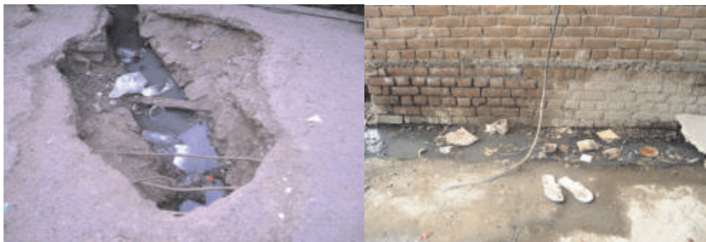
Fig.2.6 condition of drainage system
