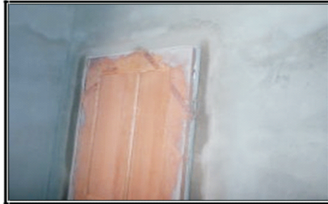
Figure 1.2. Wall of soil-cement trowed. Source: The Authors, (2017).
