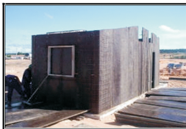
Figure 1.4. Wall in partially assembled cellular concrete. Source: The Authors, (2017).
