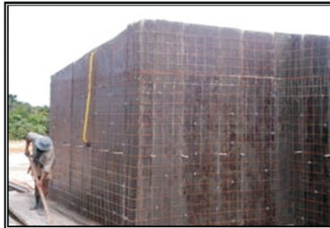
Figure 1.3. Wall in reinforced cellular concrete. Source: The Authors, (2017).
