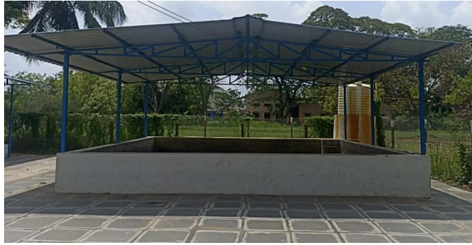
Fig 1. Solid waste management and vermicomposting concrete shed
