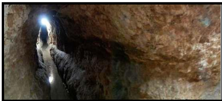
The Kharez tunnel being conserved at Naubad, Bidar.
