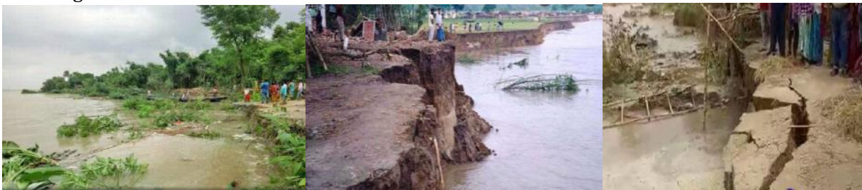
Figure No 7: River bank erosion and mass failure in Lalgola Block, Murshidabad.
